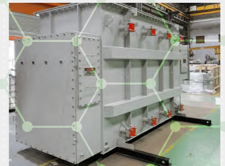
10 MVA oil-filled transformer of voltage class 27.6/13.8 kV with five-legged core design
